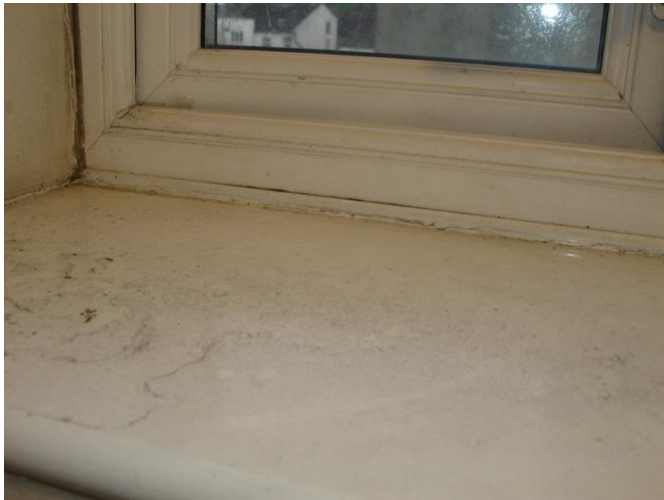
Condition of windows 2
