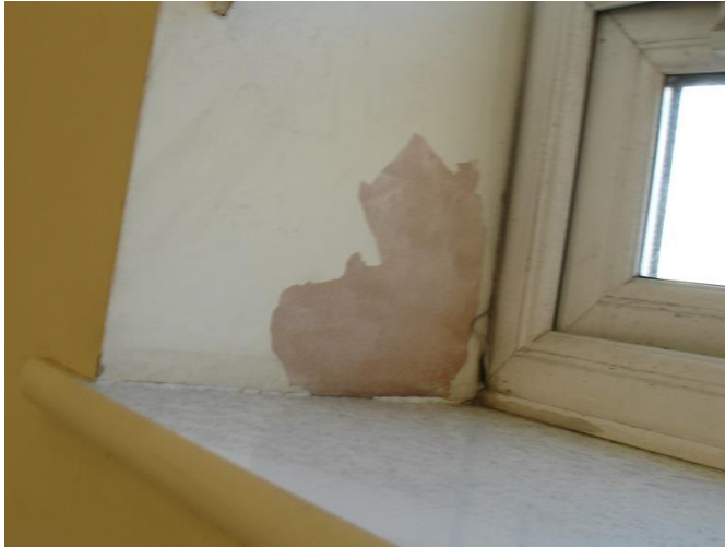
Condition of windows 1
