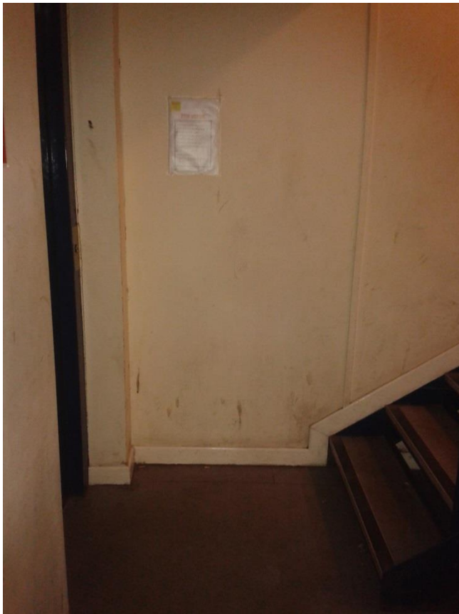
Condition of walls
