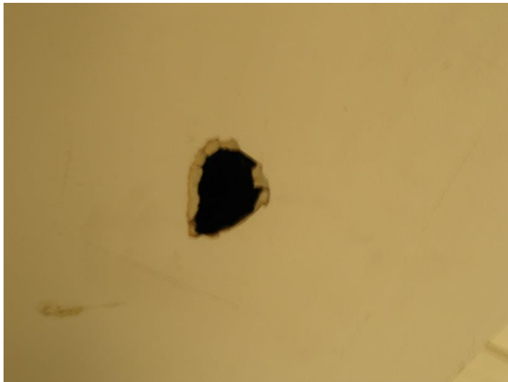
Hole punched into wall
